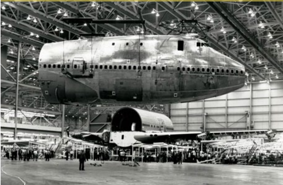
The fuselage of the first 747 began assembled in the expanded Boeing plant in Everett, Wash.
